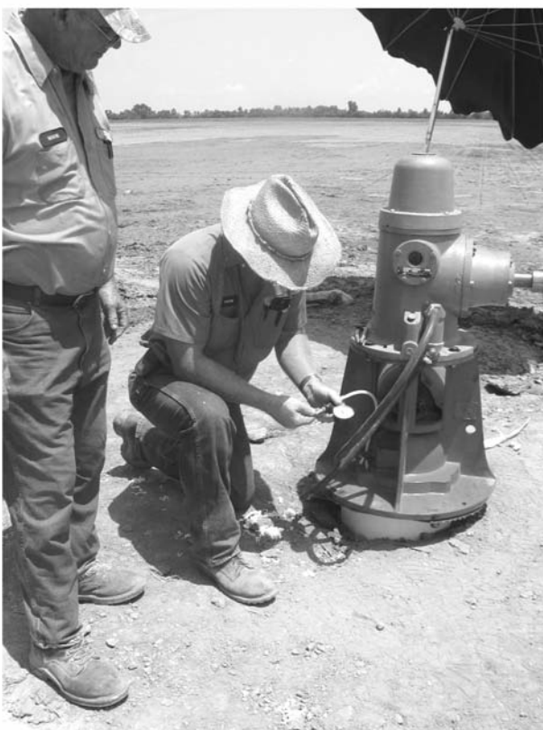
Figure 2. Water level of a newly installed pump near Portageville being read by staff from Burge Irrigation Company of Puxico, MO.
